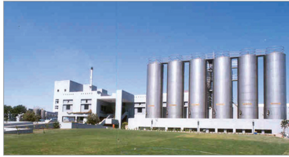
Fig. 1.3.1. Outer view of a large-size dairy processing plant
